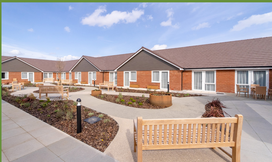
Pictured Here is Thimbleby Court Rear Garden.
